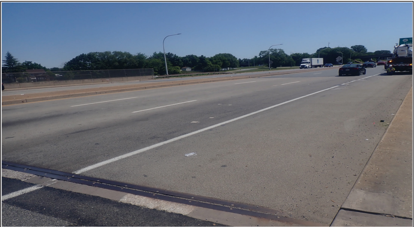
6 WEARING SURFACE LOOKING EAST IN THE EASTBOUND LANES
