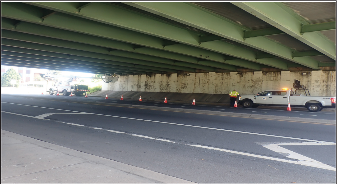
3 GENERAL VIEW LOOKING EAST
