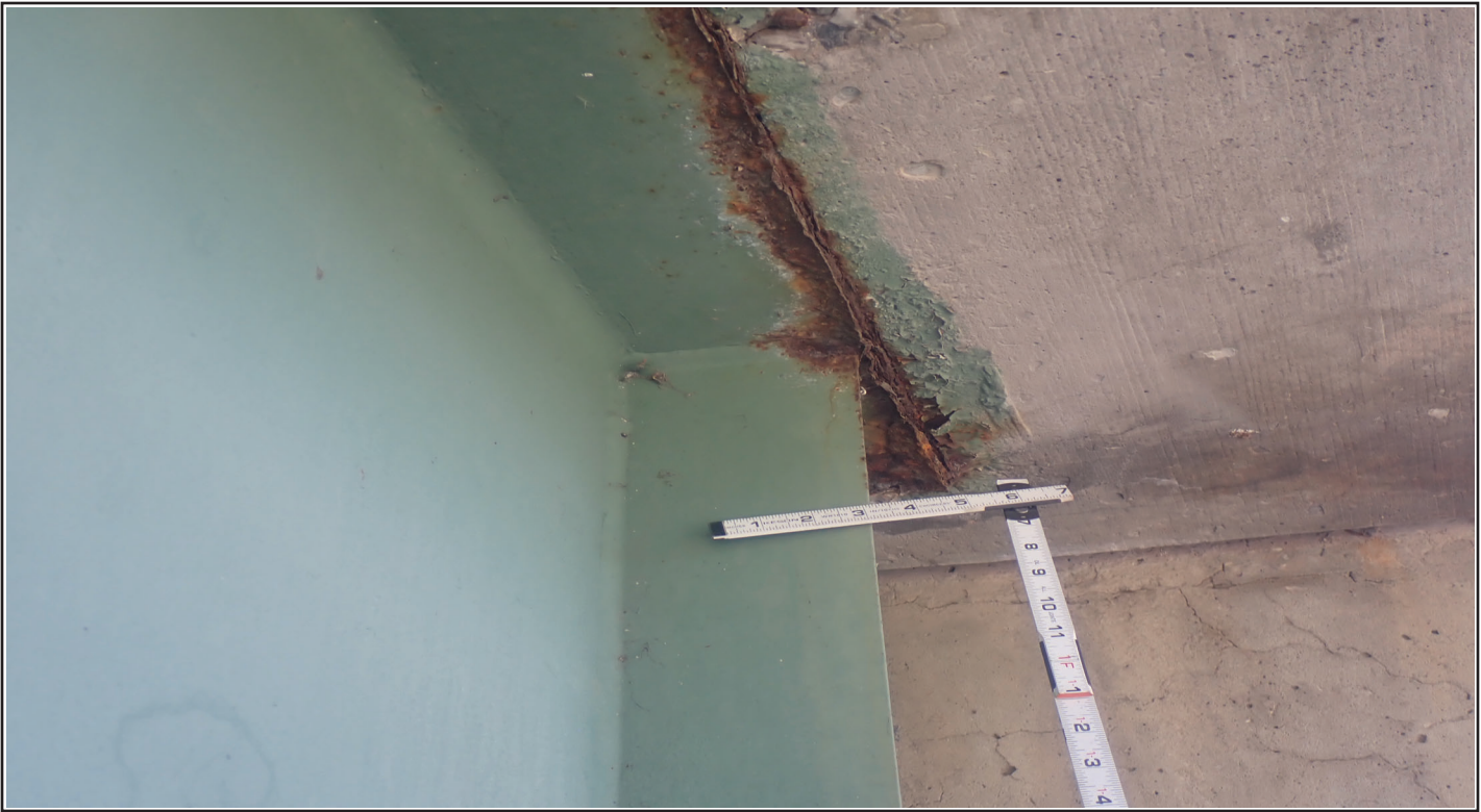
9 GIRDER 15 CORROSION w/LOSS OF SECTION TO TOP FLANGE OVER EAST ABUTMENT
